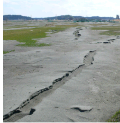
Liquefaction at Katori city near tone river during east Japan earthquake, chiba Japan.
